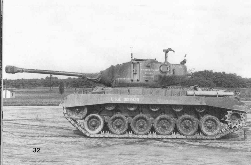
Double Baffle Muzzle Brake with No Bore Evacuator
